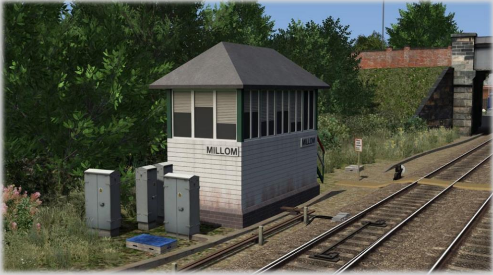
Millom Signal Box
