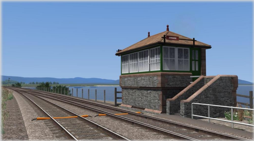
Arnside Signal Box
