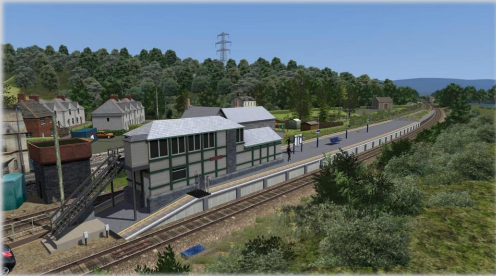
Foxfield Station & Signal Box
